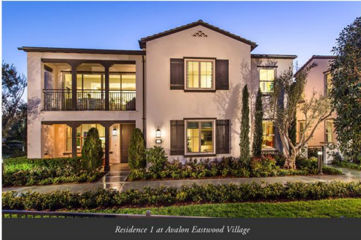
Residence 1 at Avalon Eastwood Village
